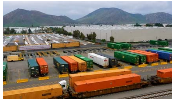
Inland Empire Intermodal Terminal Colton, California
