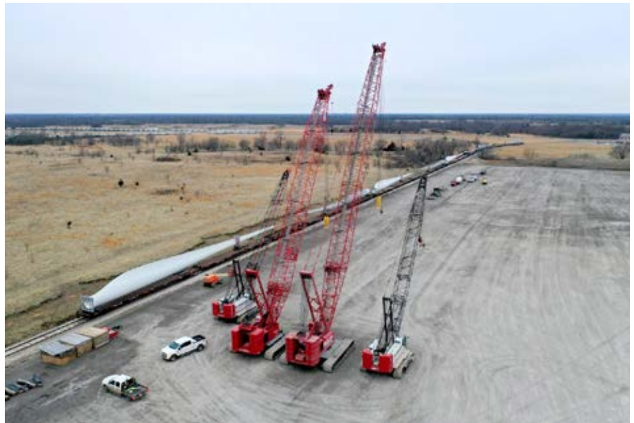
The first train in 40 years arrived at the Great Plains Industrial Park Feb.10 carrying wind turbine components.
