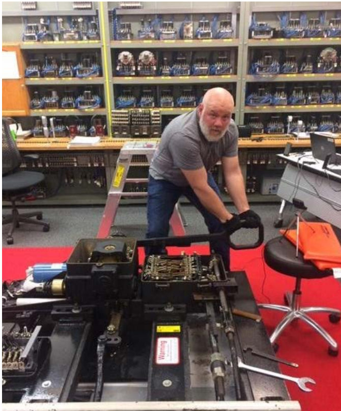
Joe Geis, senior instructor-Technical Training, Workforce Resources, demonstrates proper switch tension during a presentation at the Lone Star Training Center Signal Lab.
