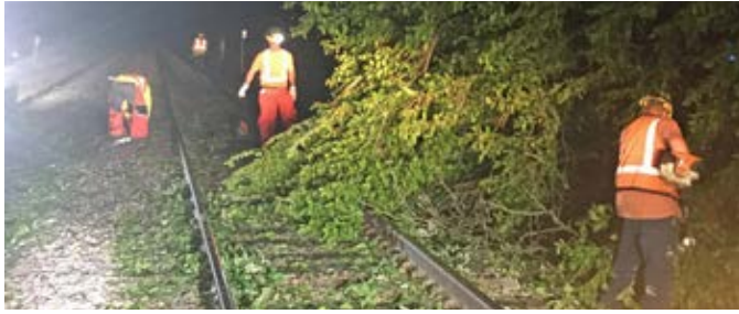
The derecho caused widespread damage across the Midwest, including in Iowa.
